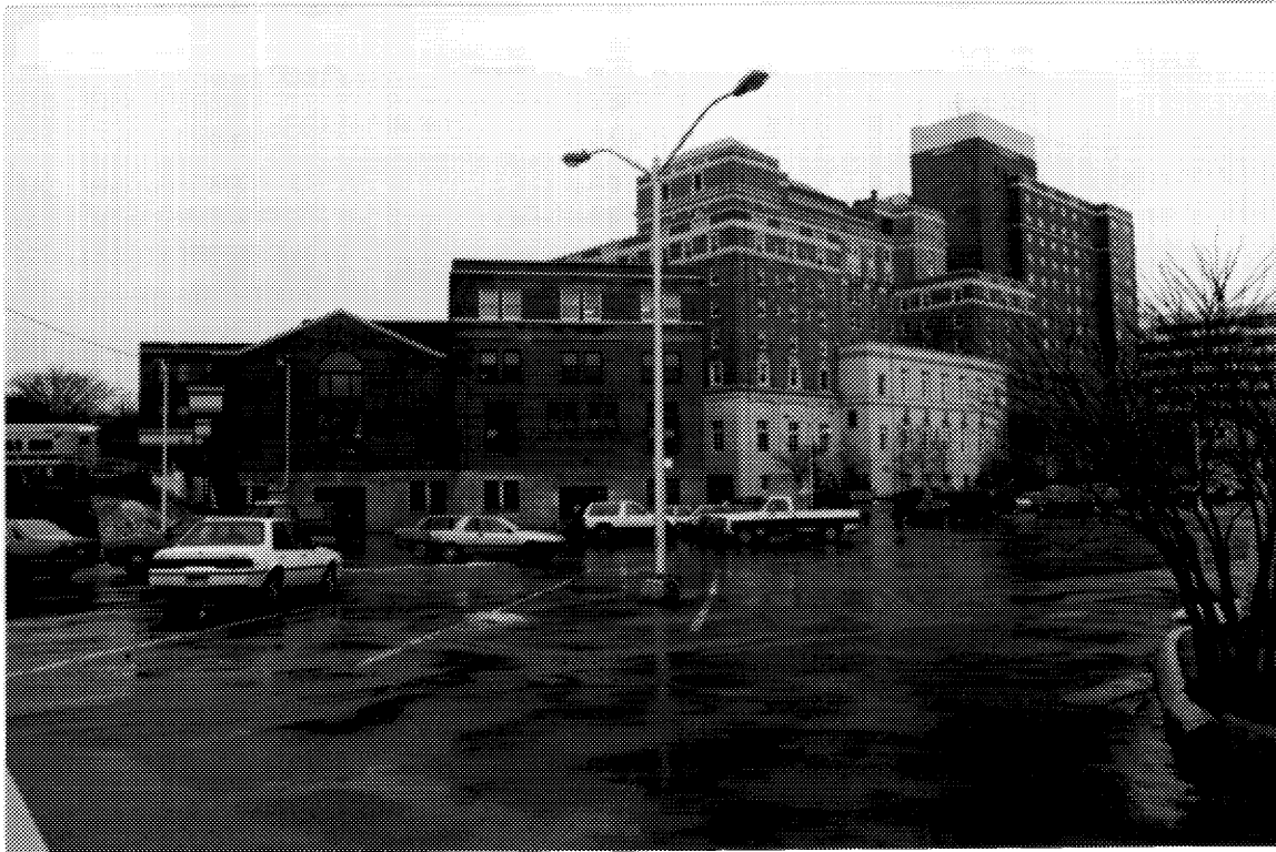
17 VIA Rail station, east elevation. ( Barry Moody, DFA, 1991. )
