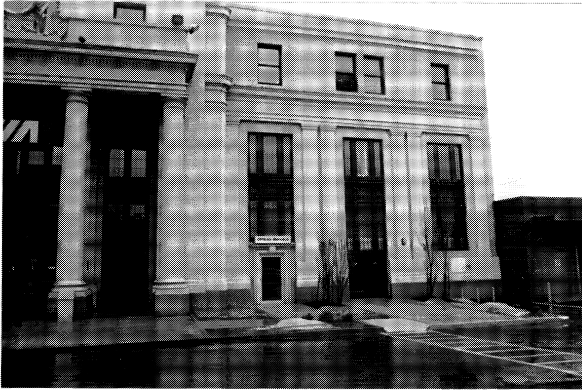
13 VIA Rail station, showing new doors (centre bay). (Barry Moody, DFA, 1991.)
