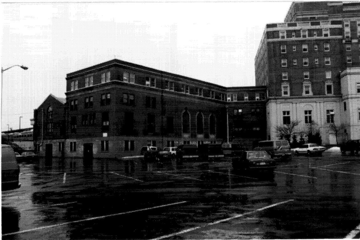
18 VIA Rail station, east and north elevations. ( Barry Moody, DFA, 1991. )
