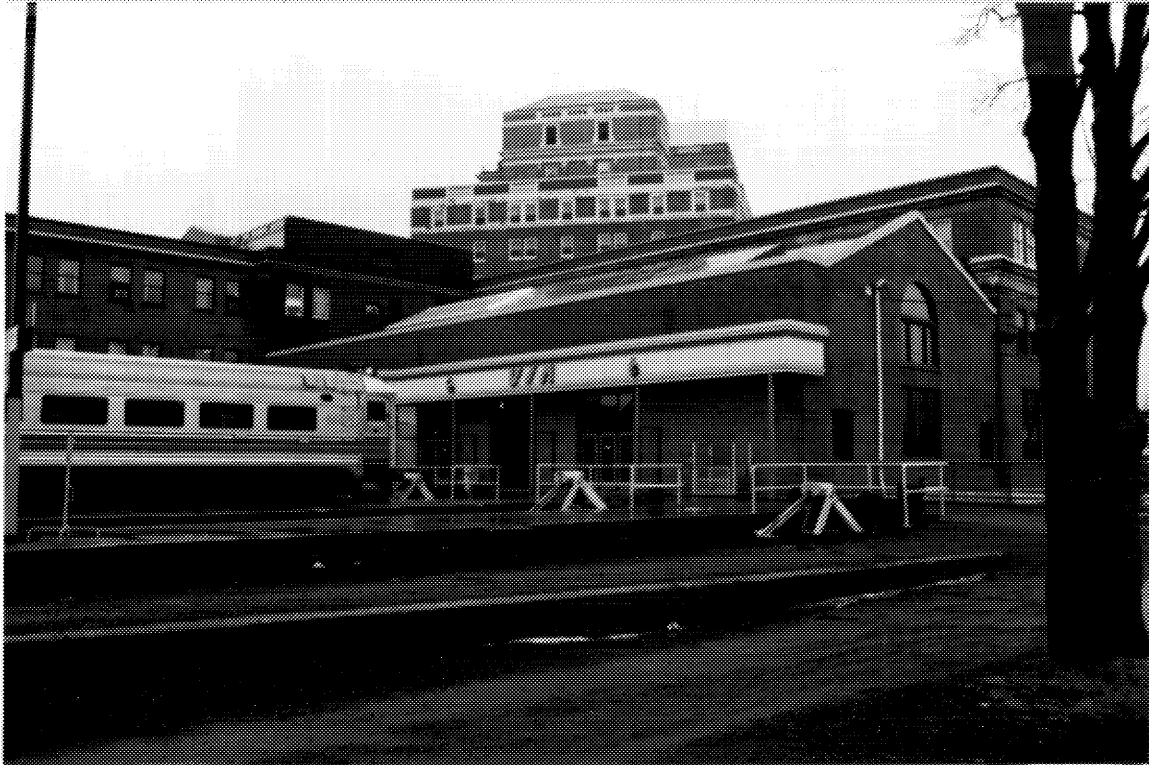
15 VIA Rail station, track-side elevation. (Barry Moody, DFA, 1991.)
