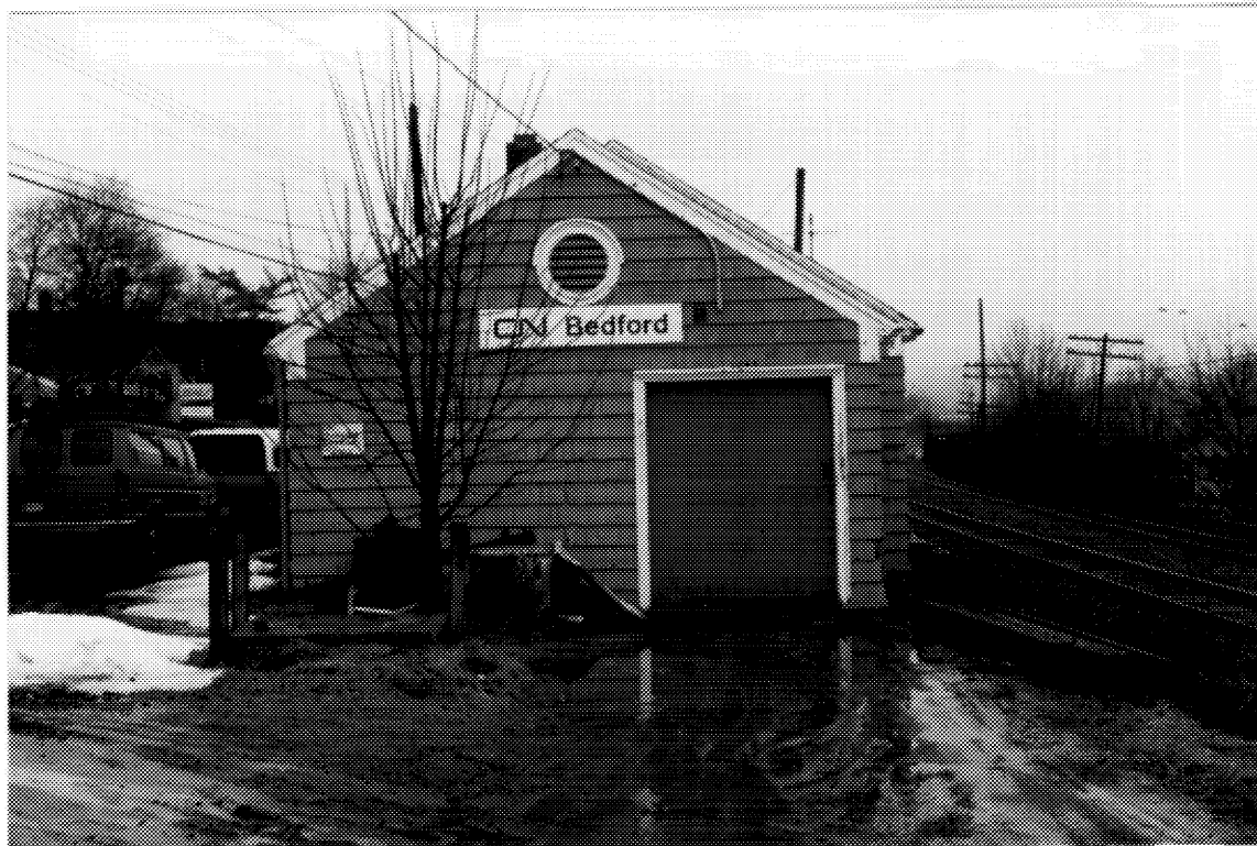
7 CNR station, showing west end modifications. ( Barry Moody, DFA, 1991. )
