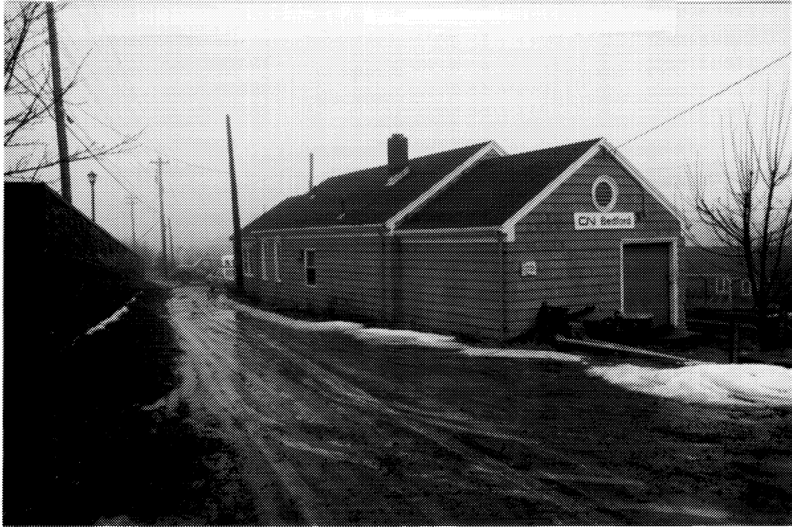
11 CNR station, road side elevation, showing contemporary window pattern. (Barry Moody, DFA, 1991.)
