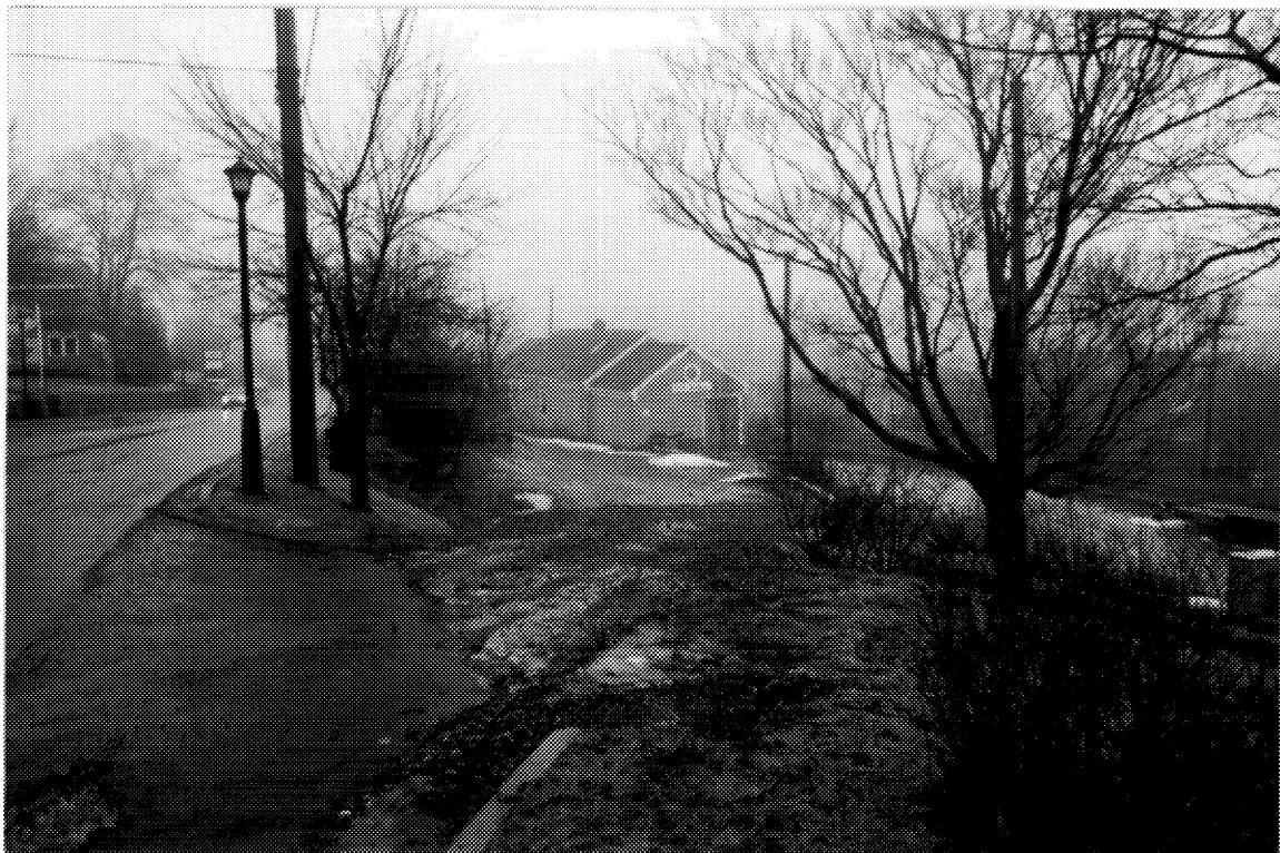
12 CNR station, showing relationship of station to highway. (Barry Moody, DFA, 1991.)
