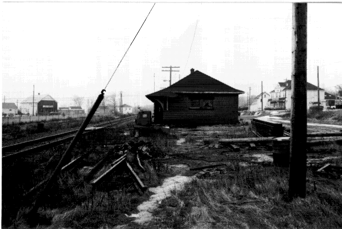
17 CNR station, exterior view from the south showing yard debris. ( Barry Moody, DFA, 1991. )
