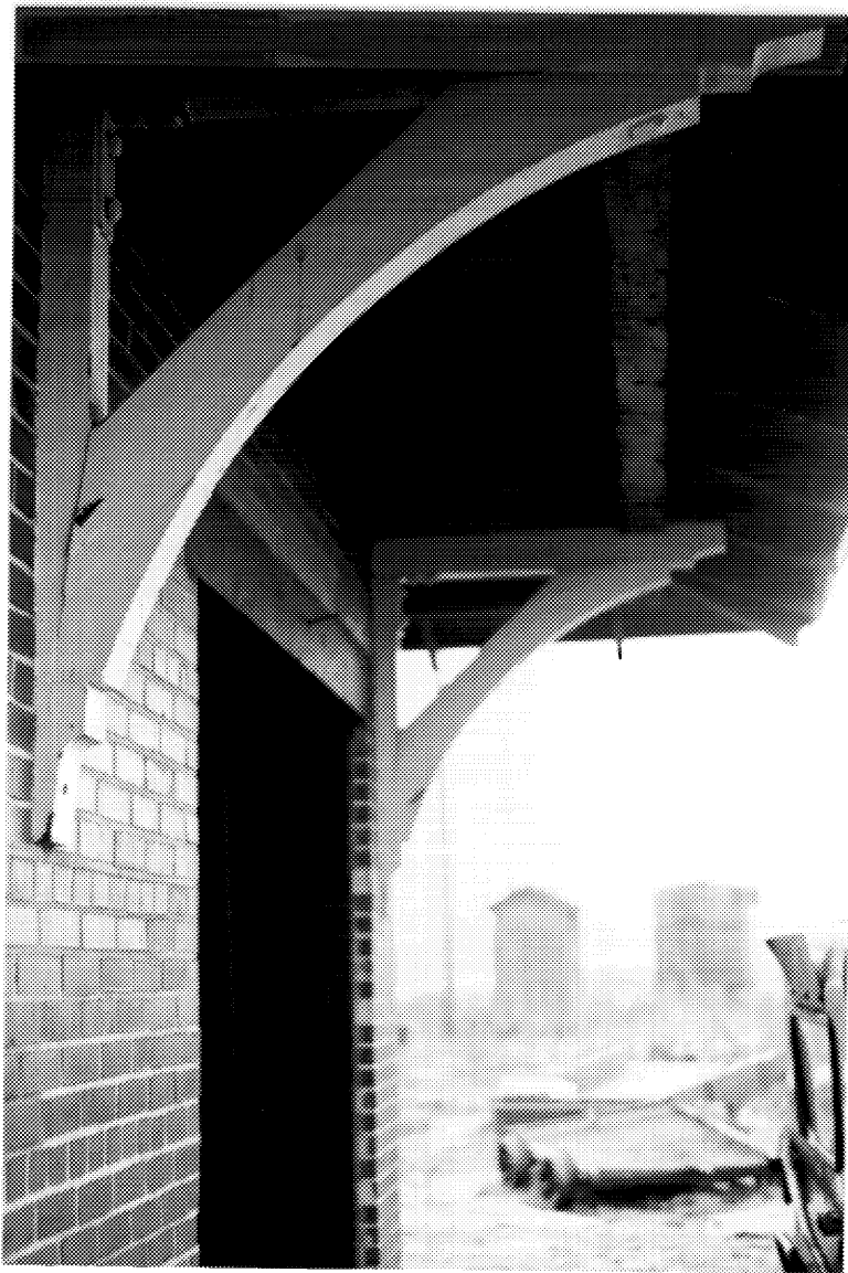
8 CNR station, wooden brackets, track elevation. ( Barry Moody, DFA, 1991. )
