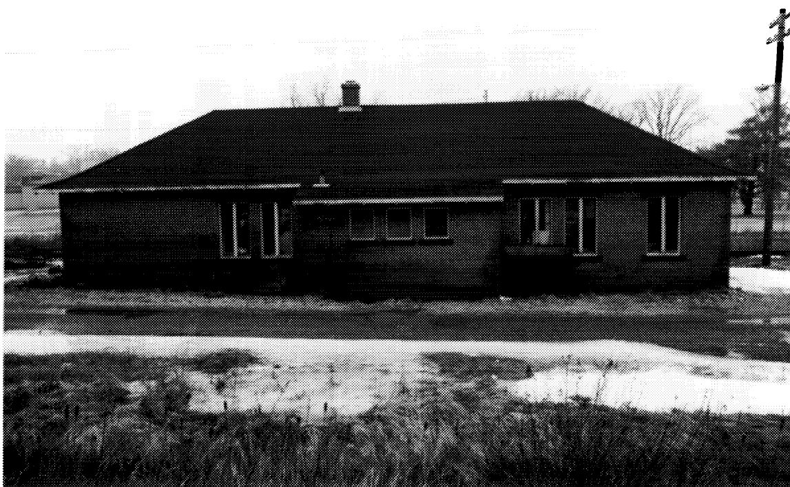
11 CNR station, street elevation. ( Barry Moody, DFA, 1991. )
