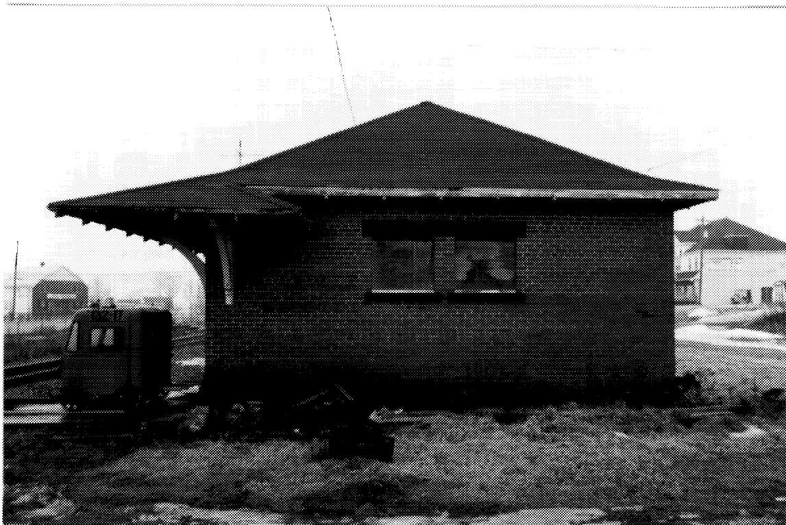
10 CNR station, south elevation. ( Barry Moody, DFA, 1991. )
