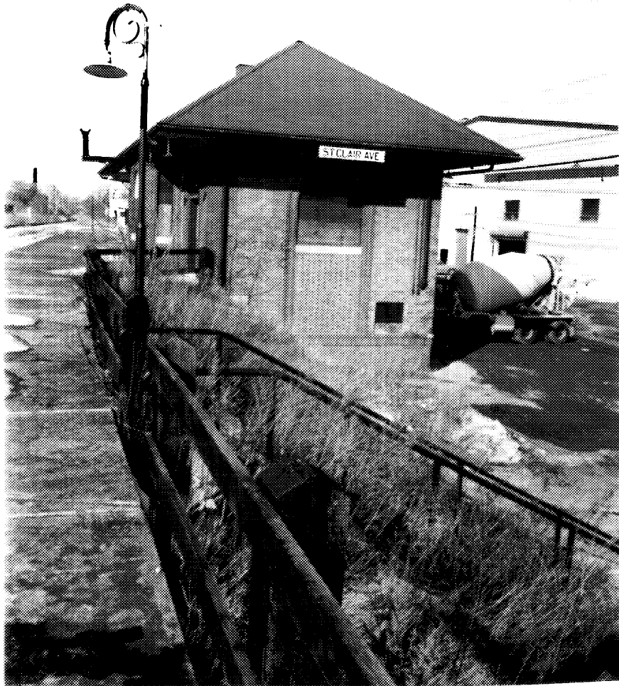
4 Former St. Clair West CNR station, south facade. ( William Dendy, 1991. )
