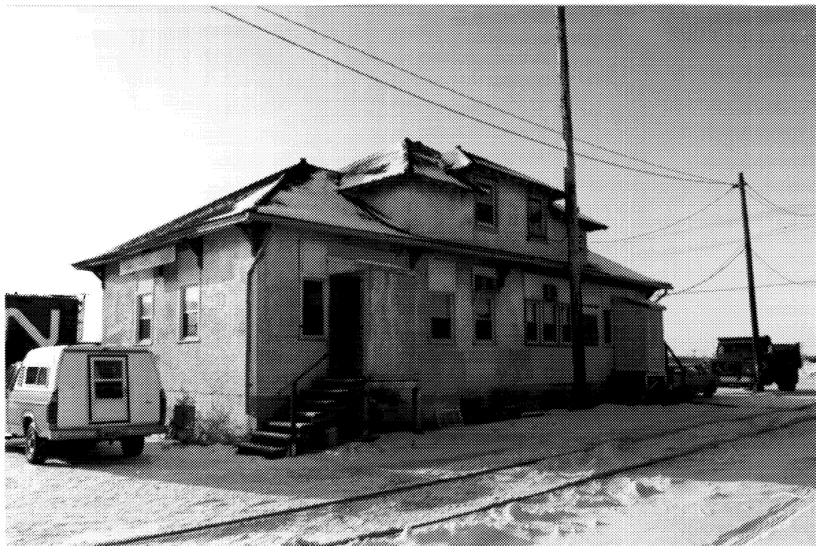
9 Former CNR station, Transcona (Winnipeg), Manitoba, north elevation and northeast corner. ( Murray Peterson, 1992. )
