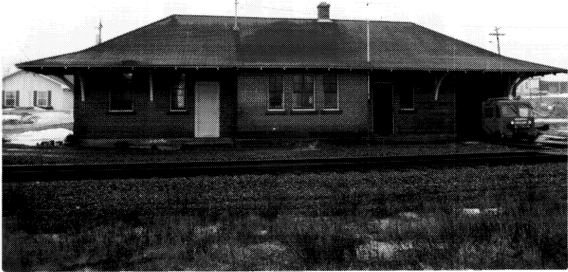
16 CNR station, Stewiacke, Nova Scotia, built 1926. ( Barry Moody, DFA, 1991. )
