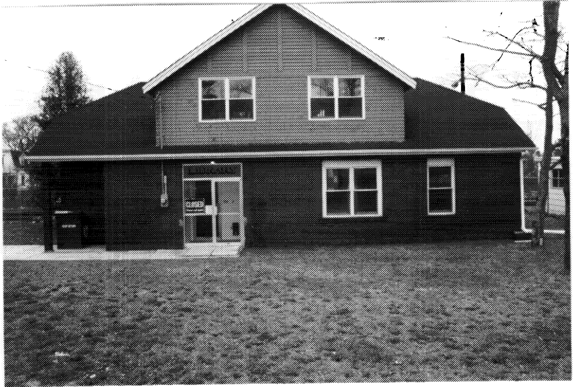
13 CNR station, street side elevation. ( Harry Jost, DFA, 1992. )
