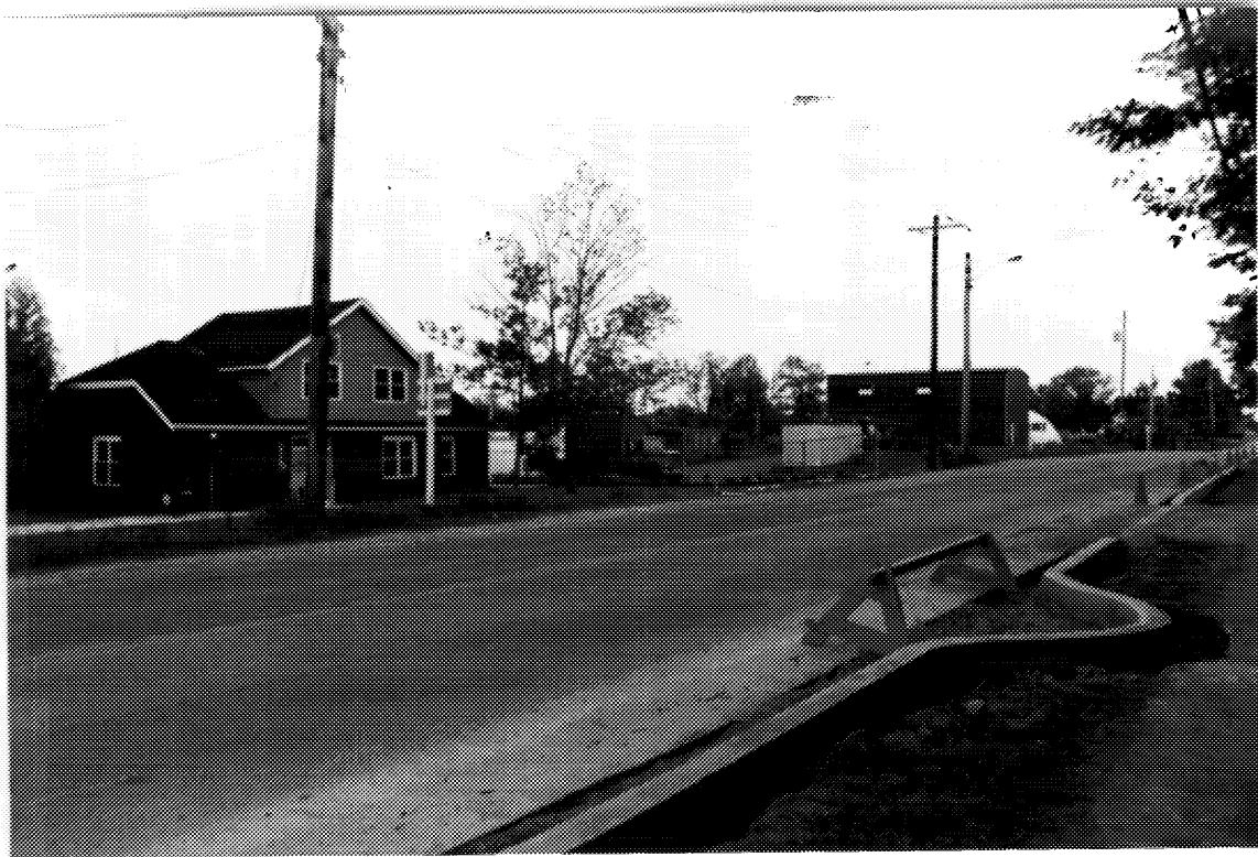
27 CNR station, showing station from adjacent highway. ( Harry Jost, DFA, 1992. )
