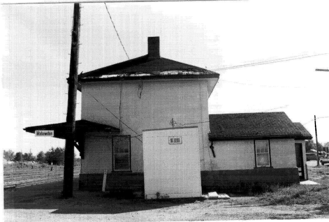
7 VIA Rail/CNR station, Wabowden, Manitoba, south end. ( Murray Peterson, 1992. )
