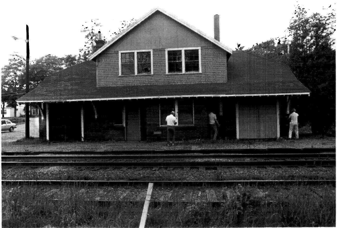
7 CNR station, track side elevation showing station prior to 1986 renovations. ( Photo courtesy of Jay Underwood, Elmsdale. )
