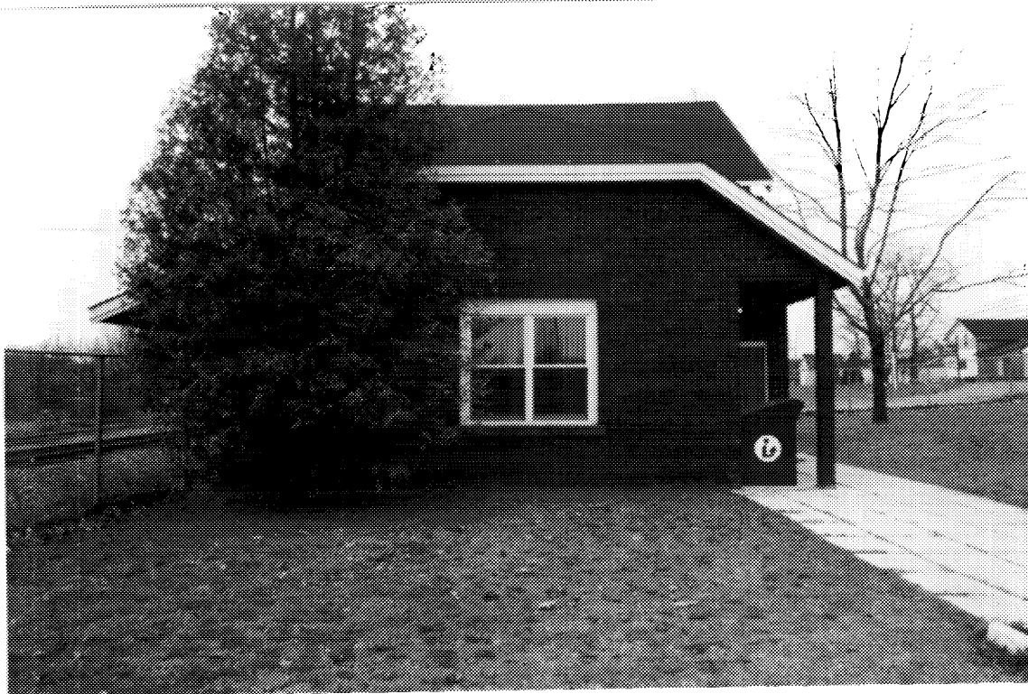
11 CNR station, end elevation. ( Harry Jost, DFA, 1992. )
