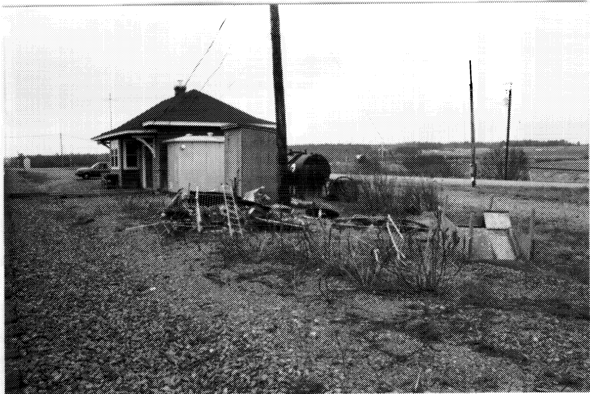
22 CNR station, debris to north of station. ( Harry Jost, DFA, 1992. )
