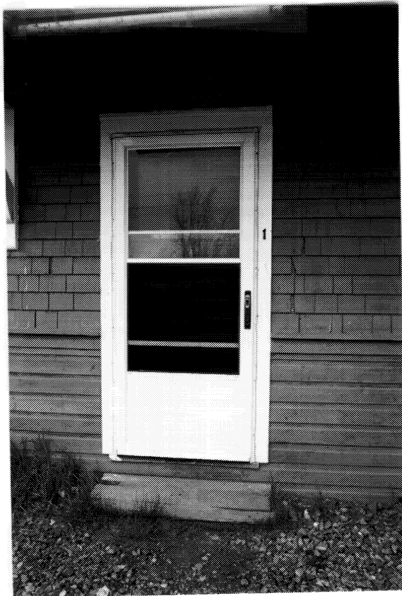
12 CNR station, detail showing aluminum entry door, track side elevation. (Harry Jost, DFA, 1992.)
