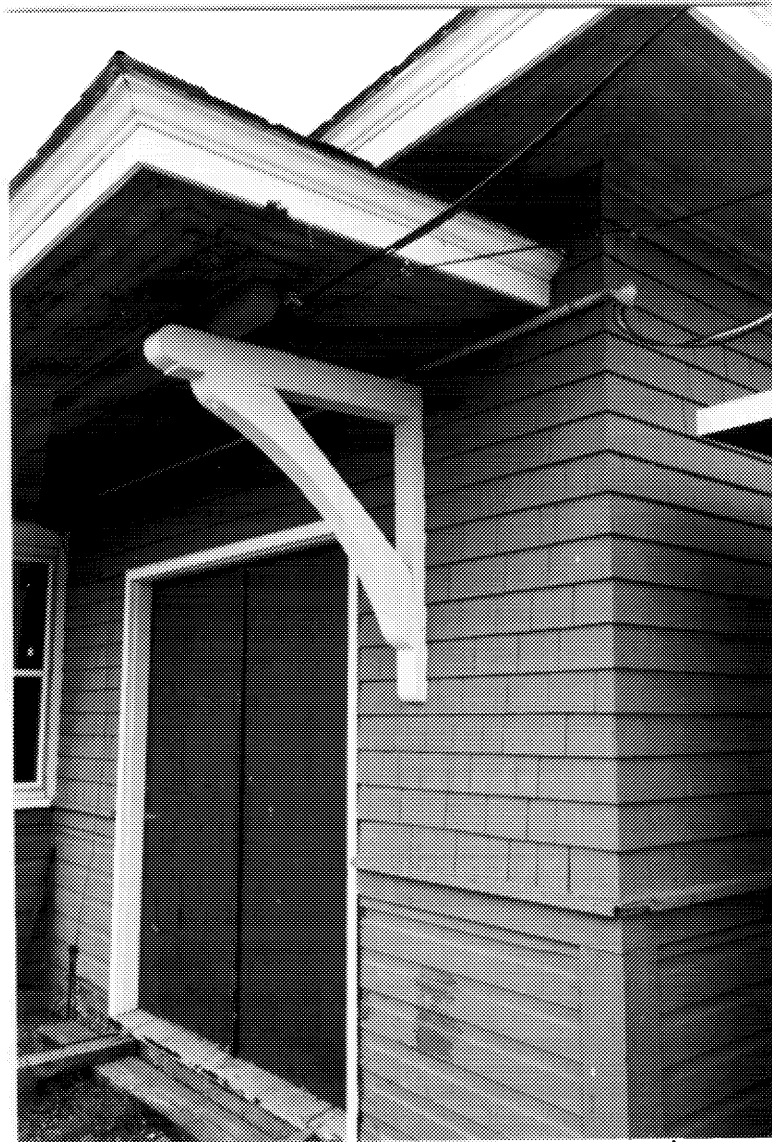
8 CNR station, detail showing bracket, track side elevation. ( Harry Jost, DFA, 1992. )
