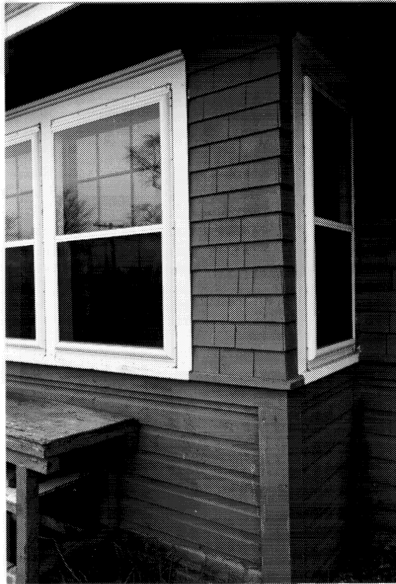
7 CNR station, detail showing siding, track side elevation. ( Harry Jost, DFA, 1992. )
