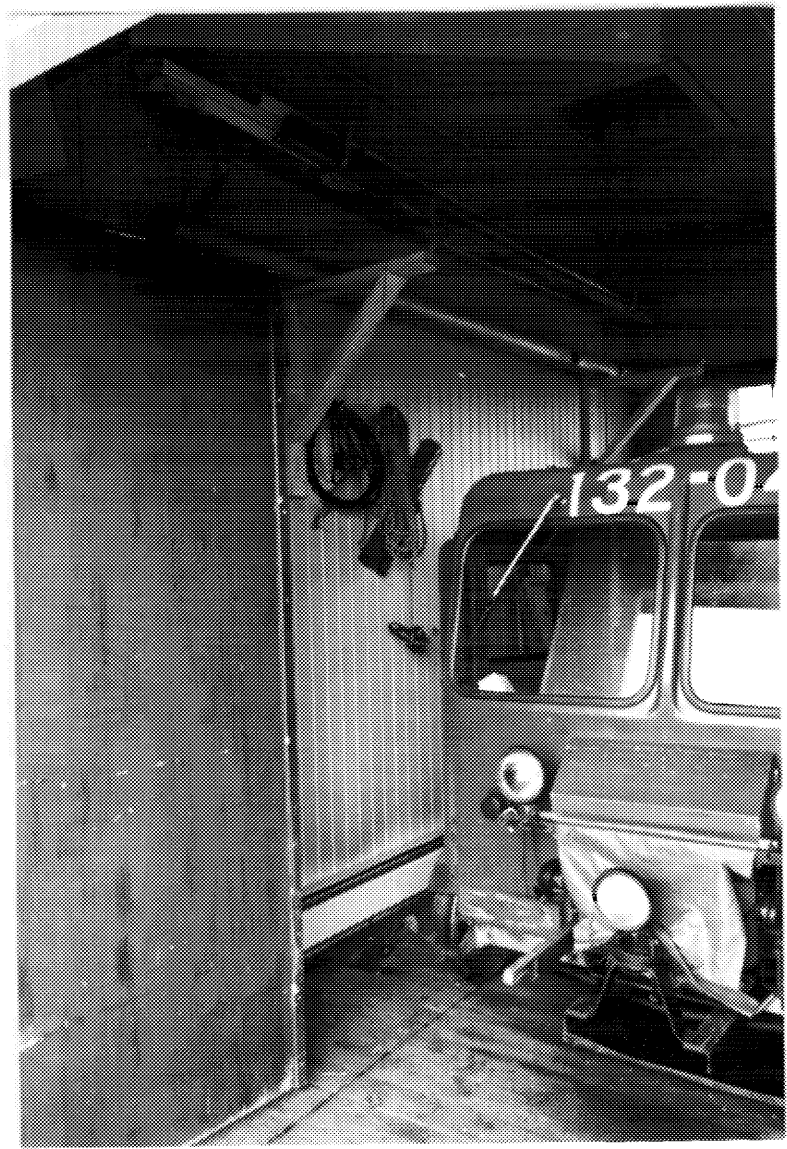
14 CNR station, detail showing tongue and groove finish. ( Harry Jost, DFA, 1992. )
