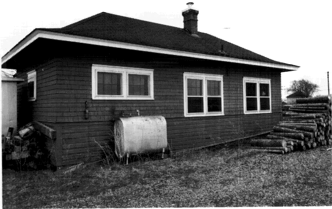
9 CNR station, rear elevation. ( Harry Jost, DFA, 1992. )
