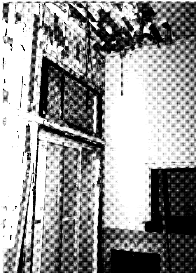
14 CNR West Toronto station, corner of room in north half. ( HRSD files, 1992. )
