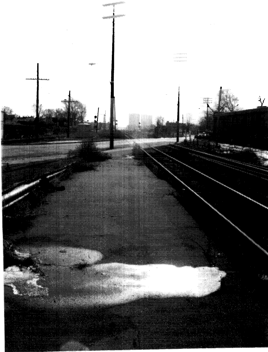
16 View looking south from the CNR West Toronto station, with tracks on both sides. ( HRSD files, 1991. )
