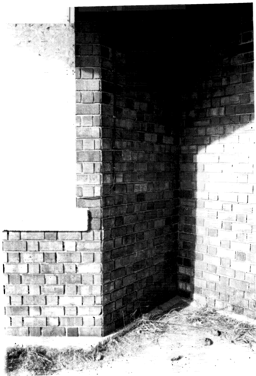
9 CNR West Toronto station, detail of masonry on south bay. (HRSD files, 1991.)
