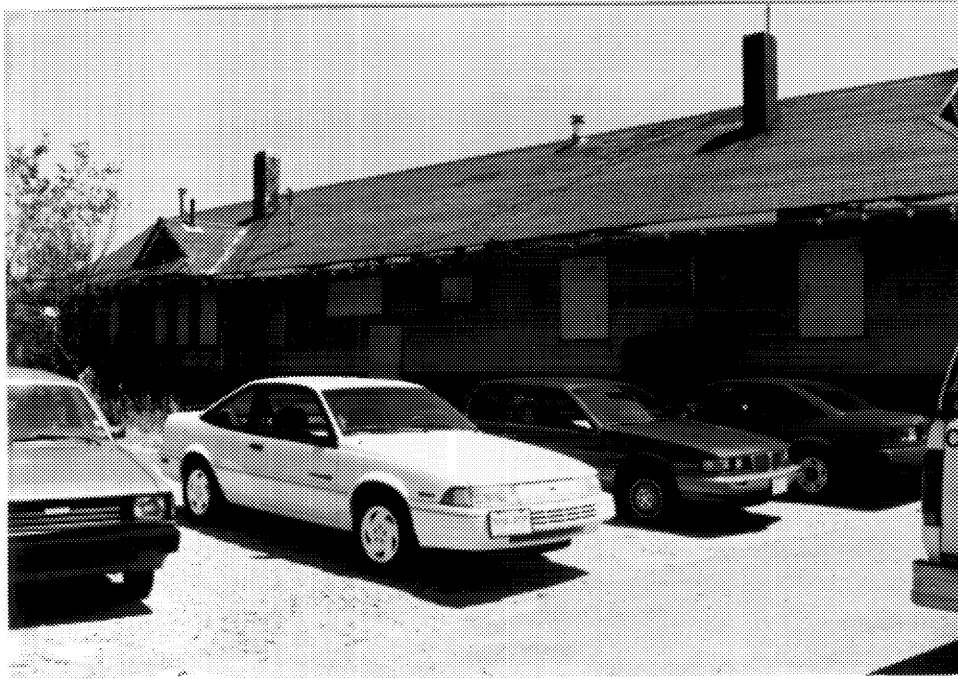
13 CNR station, Mimico, north elevation. The little gable at the left indicates the lavatories. ( HRSD files, 1991. )
