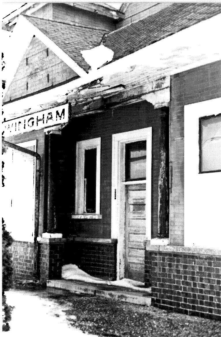
11 The front door of the Wingham station. (M. Carter, 1992.)
