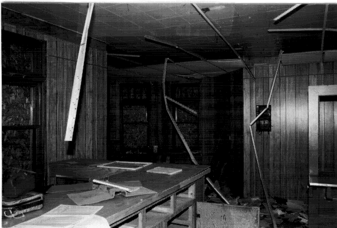
8 Former CNR/VIA Rail station, Oba, Ontario, office/ticket counter area. ( Murray Peterson, 1992. )
