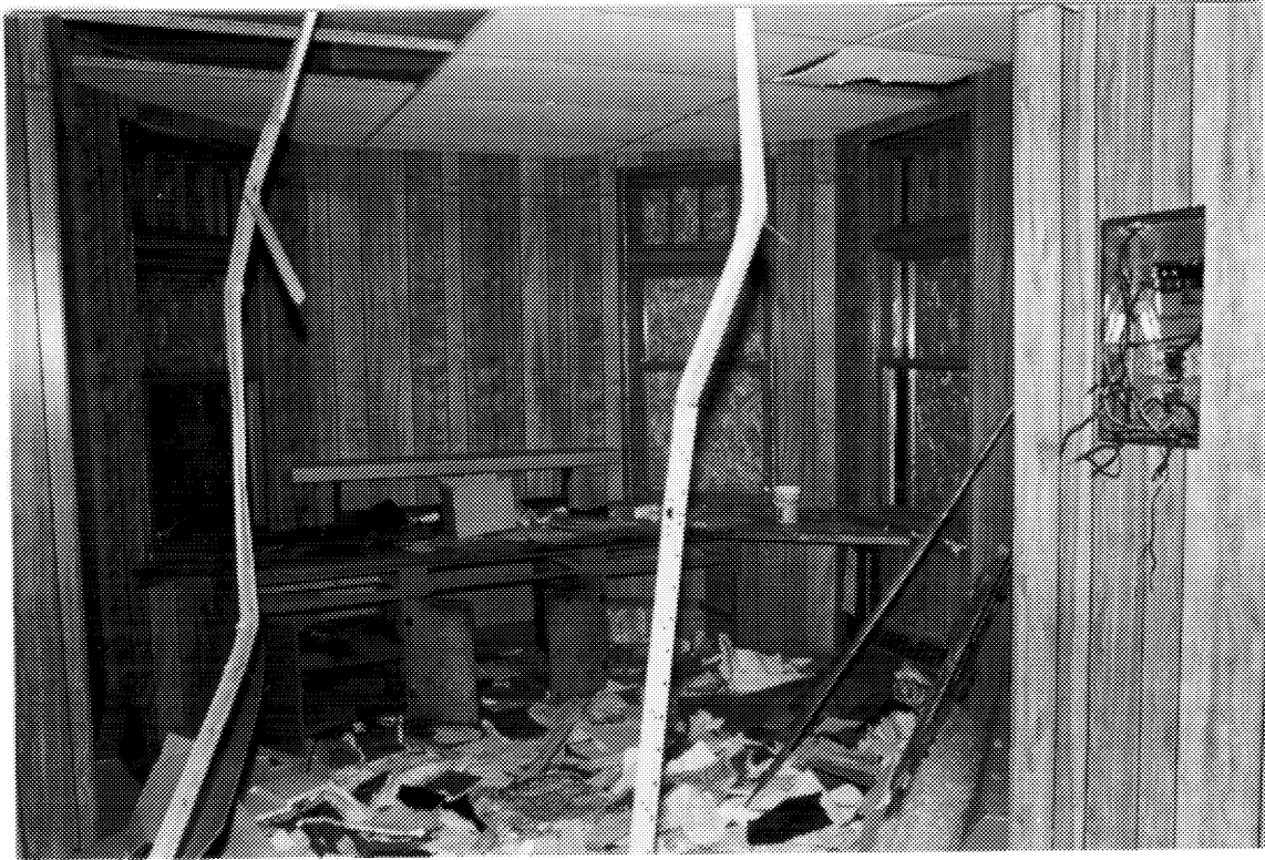
9 Former CNR/VIA Rail station, Oba, Ontario, first floor bay window. ( Murray Peterson, 1992. )
