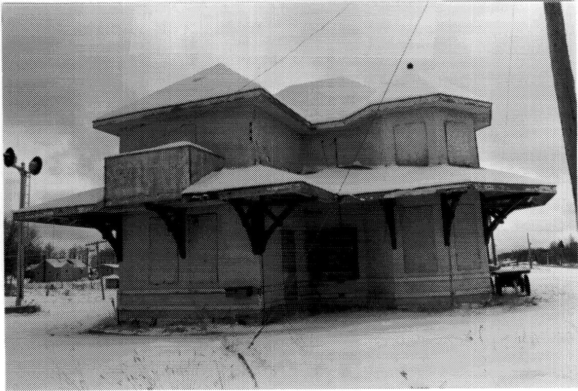
6 Former CNR/VIA Rail station, Oba, Ontario, west end. ( Murray Peterson, 1992. )
