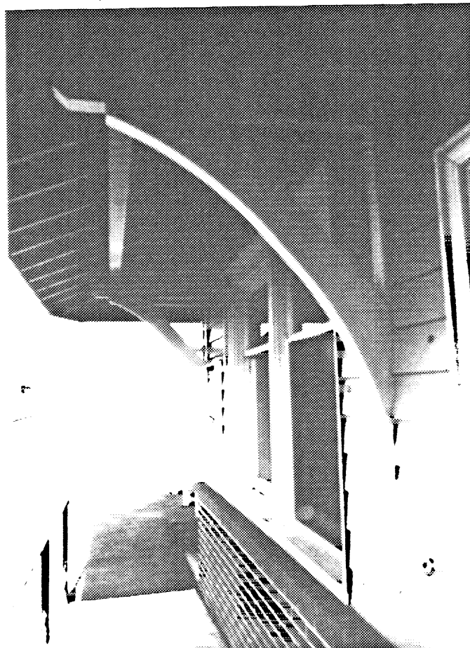
11 CNR station, Rogersville, showing plain wooden brackets with unchamfered edges. ( Robert Power, 1992. )
