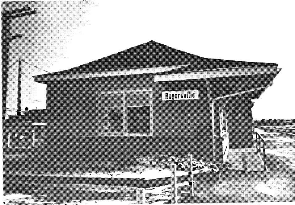
10 CNR station, Rogersville, north elevation, showing wrap-around eaves. ( Gwen Martin, 1992. )
