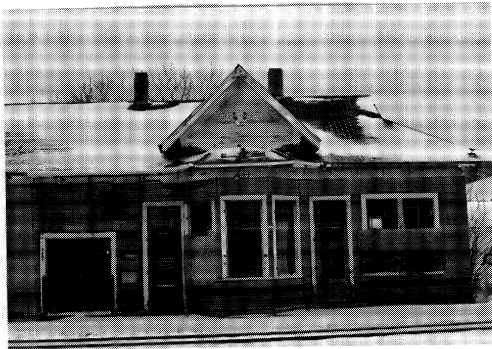
12 North end, east facade, South River CNR station. ( M. Carter, Heritage Research Associates, 1993. )
