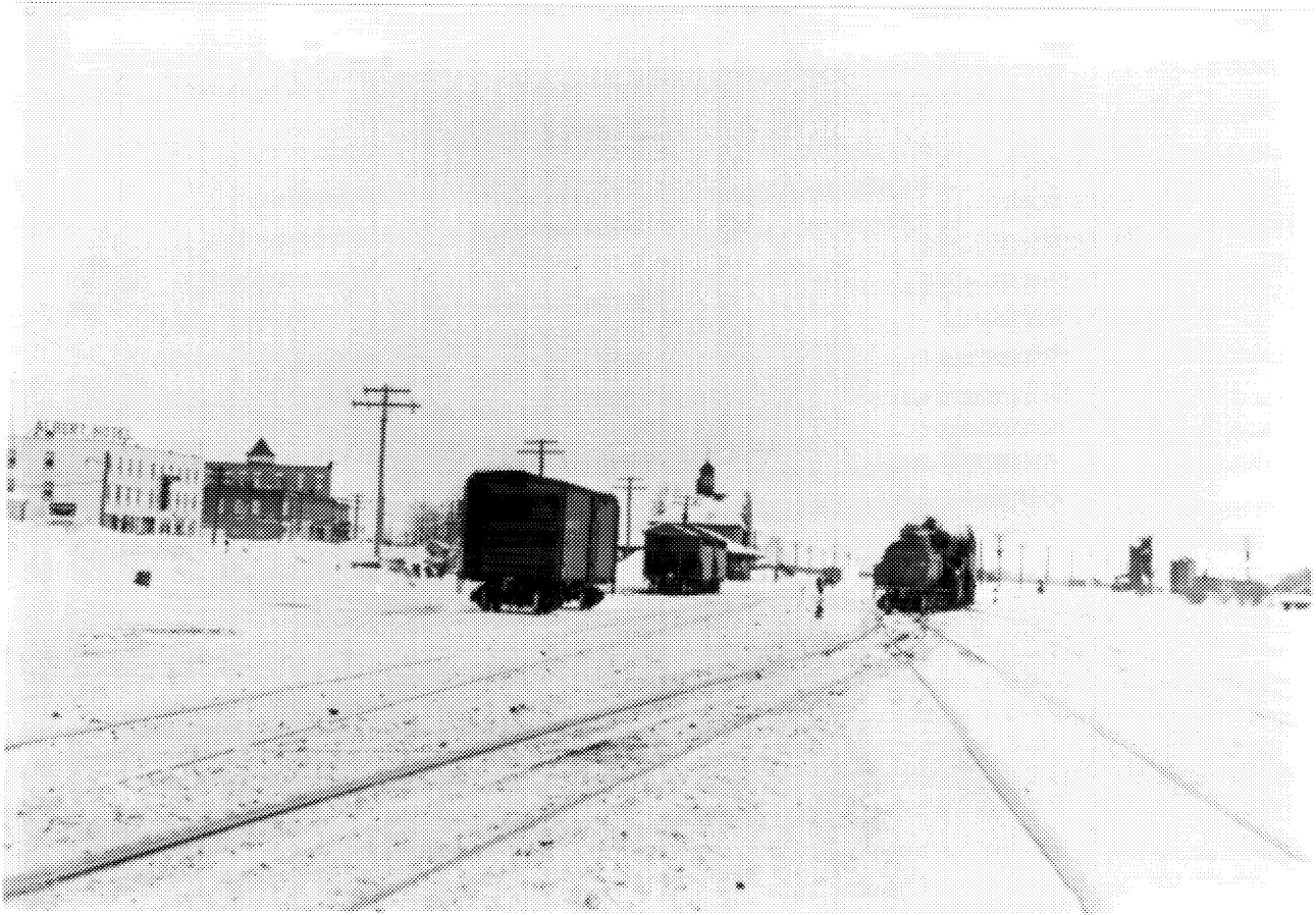
26 Cochrane, Ontario; yards, T&NO round house, water tower and coal chute in right background, NTR facilities left of T&NO facilities (not pictured), n.d. ( Courtesy of Dave Rudyk, Cochrane. )
