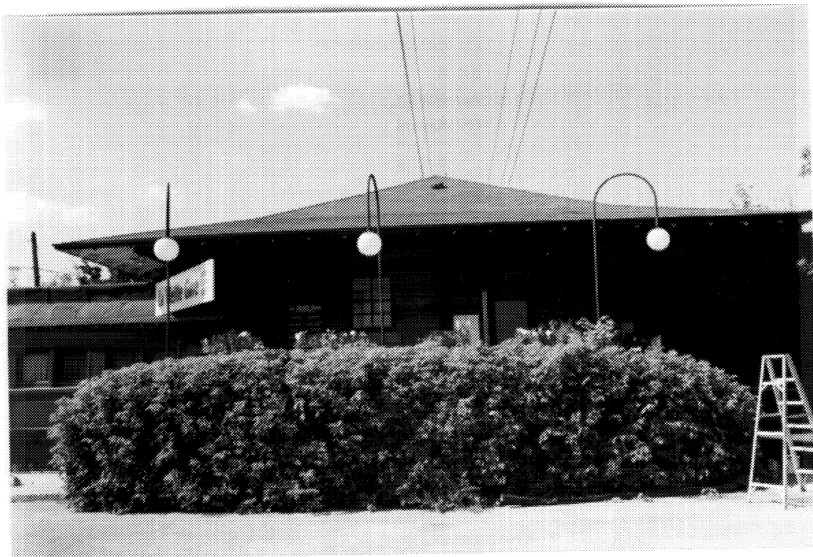
17 Former CNR station, St. Boniface, Manitoba; south elevation. ( Murray Peterson, 1993. )
