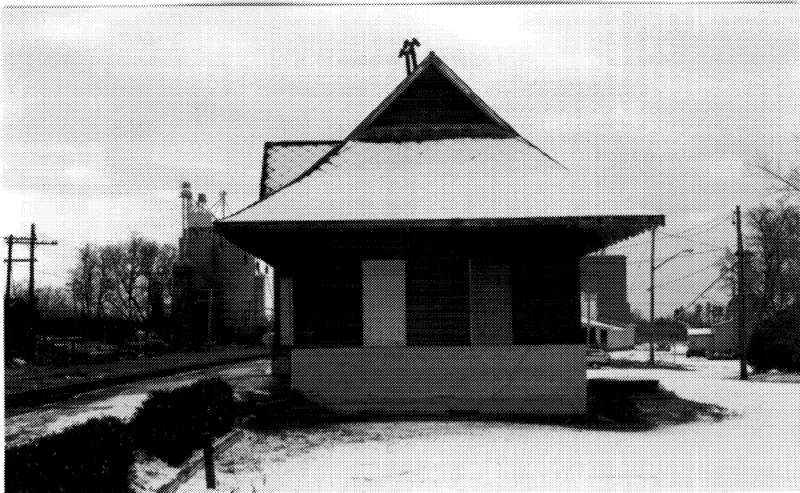
10 East elevation of the Maxville station. ( Nancy Fairbairn, Heritage Research Associates, 1992. )
