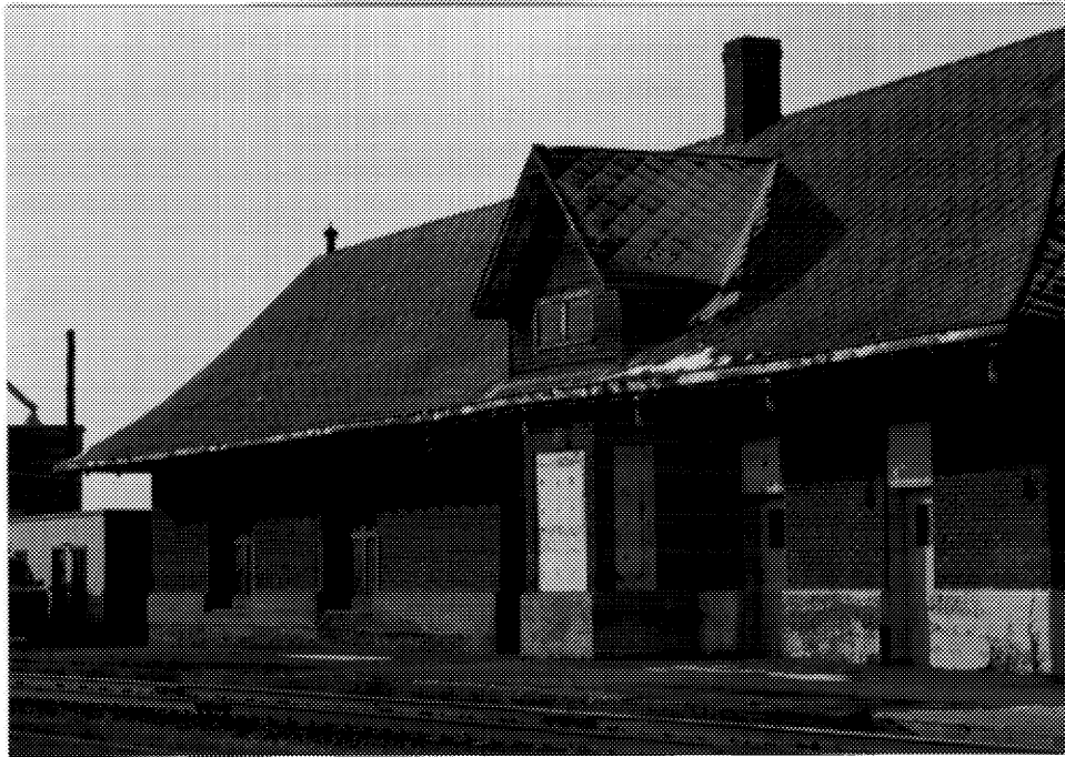
15 Bay and gable combination, Maxville GTR station. ( Nancy Fairbairn, Heritage Research Associates, 1992. )
