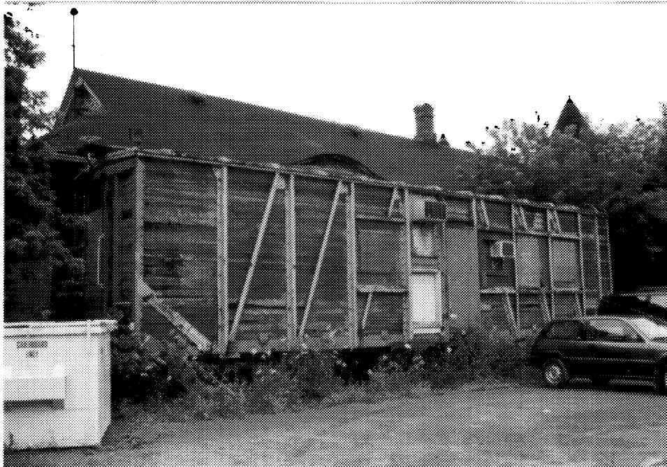
12 Grimsby station, rail car added to south back. (A. M. de Fort-Menares, 1993.)
