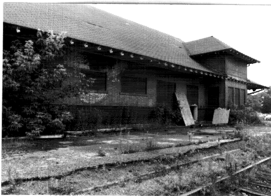
8 Port Colborne station north side. ( A. M. de Fort-Menares, 1993. )
