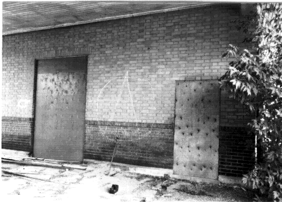
18 Breezeway doors from baggage room. ( A. M. de Fort-Menares, 1993. )
