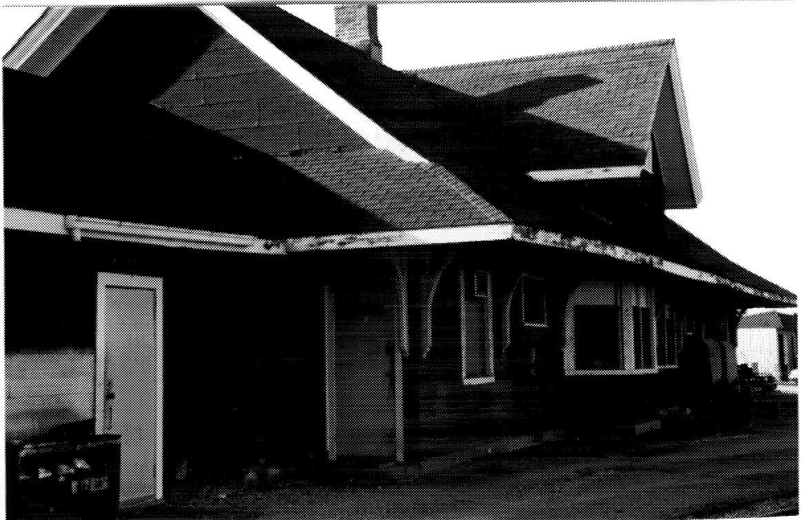
19 CNR station, Merritton, north side elevation, three quarter view from the northeast, detail showing weathered condition of roof tiles on the cross-gable, and general condition of the roof and siding. ( John L. Nicholls, Analytica Associates, 1993. )
