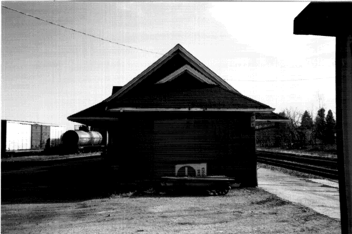
17 CNR station, Merritton, west end elevation, showing characteristic profile of gabled hip roofs over the enclosed canopied shelter, now clad in grey-painted plywood. ( John L. Nicholls, Analytica Associates, 1993. )
