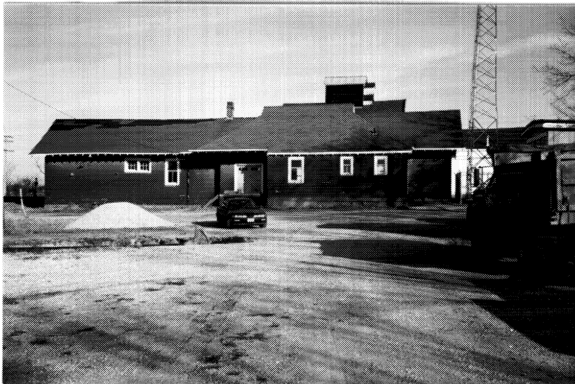
13 CNR station, Caledonia, south elevation, showing the effect of the 1924 extension of the building by some 20 feet at the west or freight end. (John L. Nicholls, Analytica Associates, 1993.)
