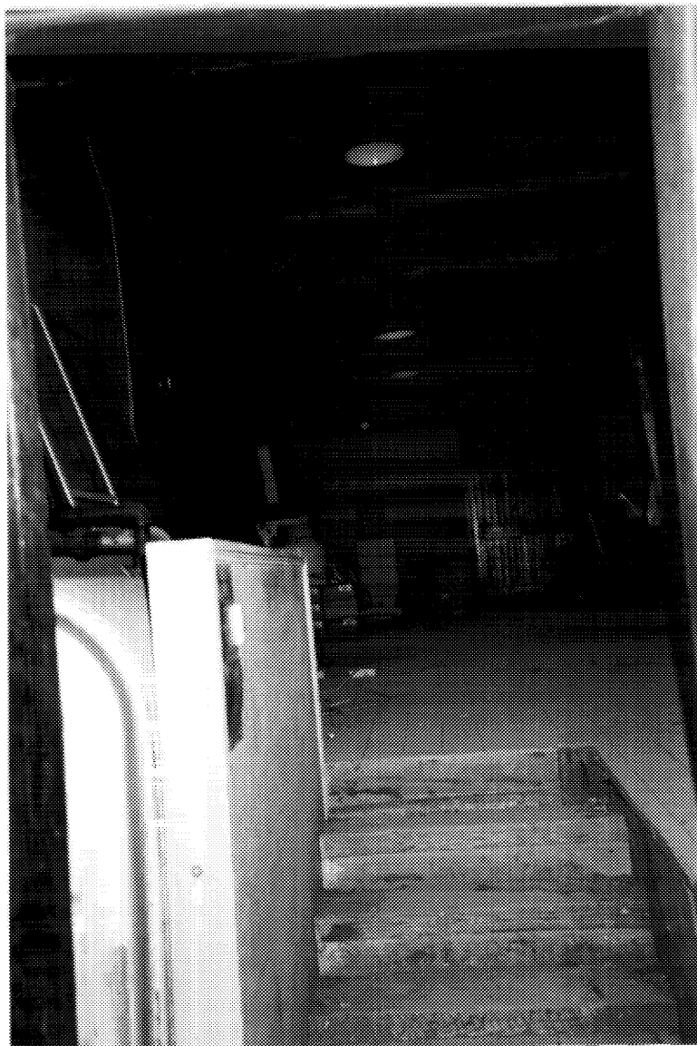
19 CNR station, Bradford, interior; detail of the original freight room at the north end of the building, showing the raised floor which facilitated direct loading and unloading of rail cars from the raised platforms. ( John L. Nicholls, Analytica Associates, 1993. )
