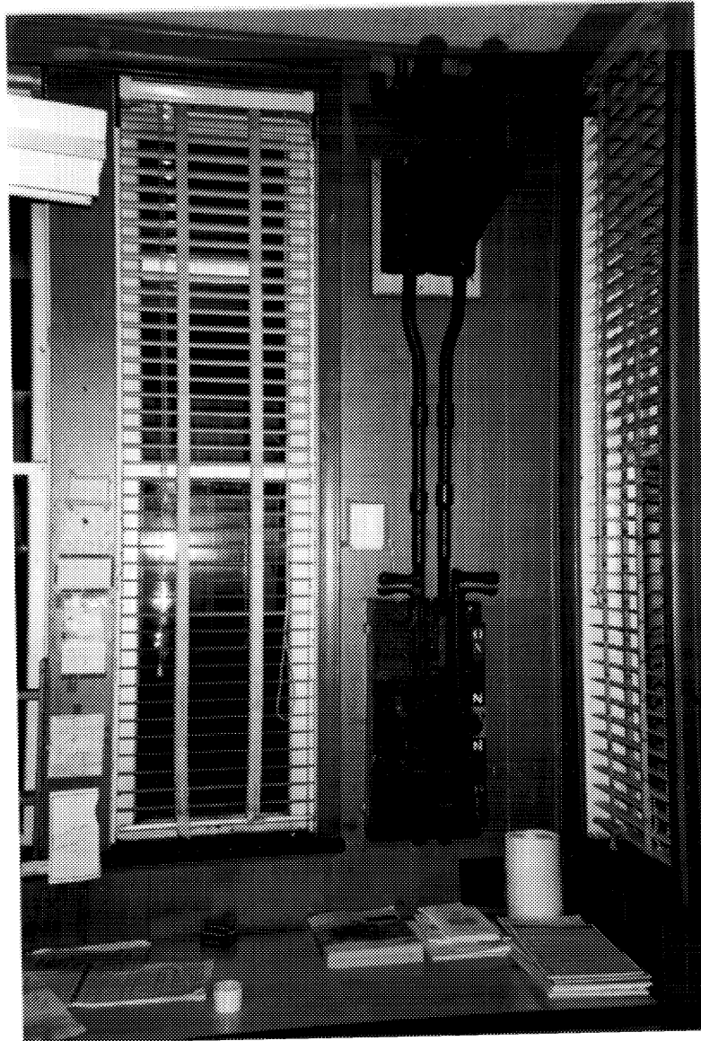
20 CNR station, Bradford, interior; detail of the track side bay, showing the operator's traditional vantage point, with a clear view up and down the line, manual signal switch, and modern panelling. ( John L. Nicholls, Analytica Associates, 1993. )
