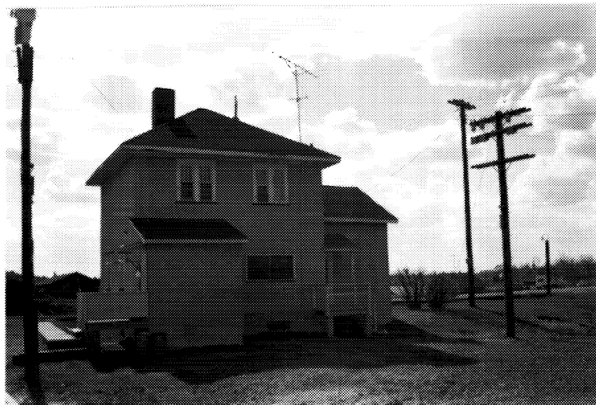
27 Rear, Field station, 1973. This photo shows the porches on the west and north sides that have since disappeared. ( CIHB, 06014800000001. )
