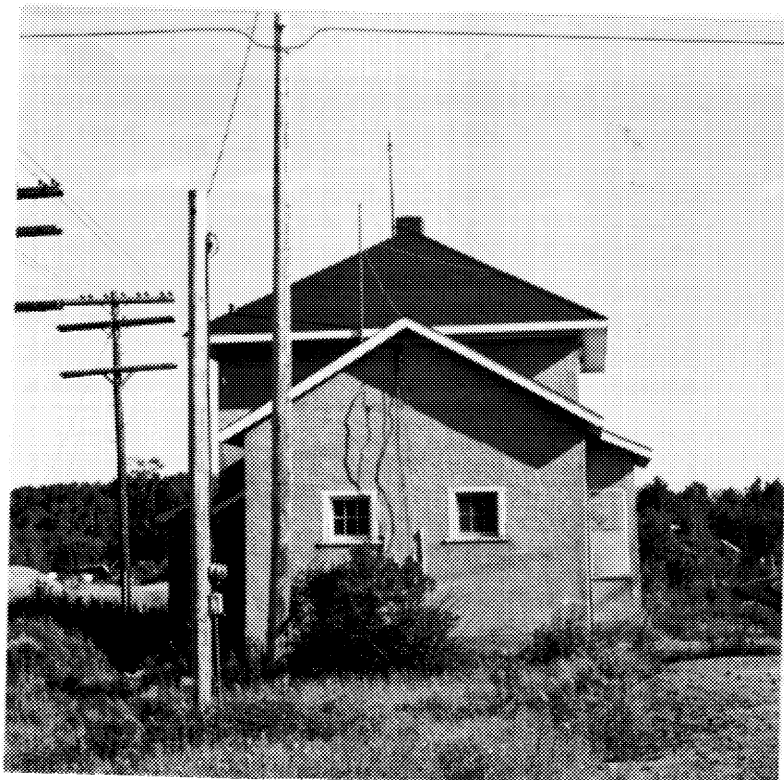
12 West facade, Field station. ( M. Carter, Heritage Research Associates, 1994. )
