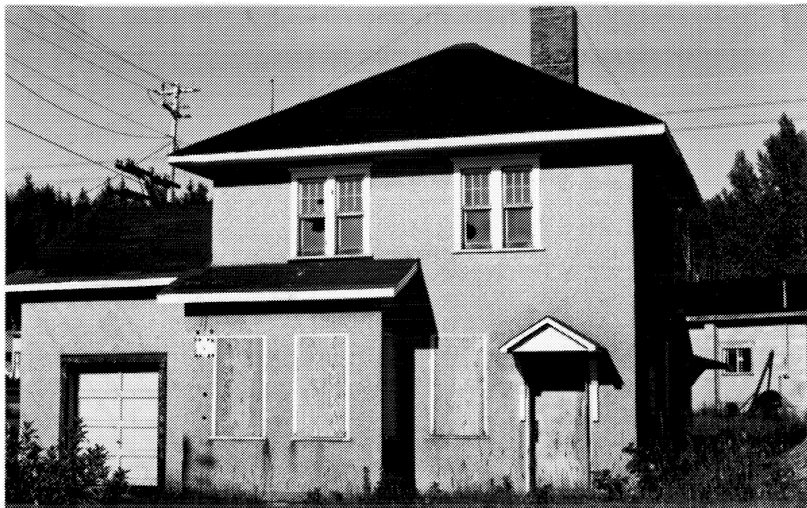
9 South (track) facade, Field station. (M. Carter, Heritage Research Associates, 1994.)
