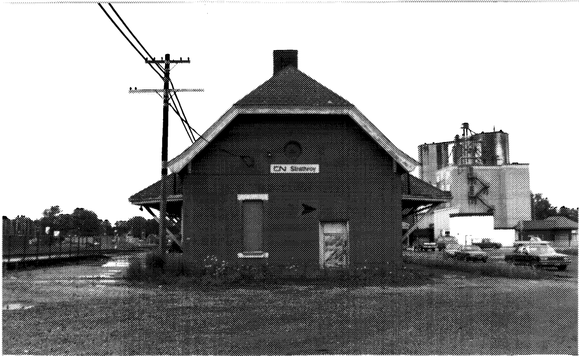
7 Strathroy station, east gable end with rebuilt opening. (Historica Research Limited, August 1992.)
