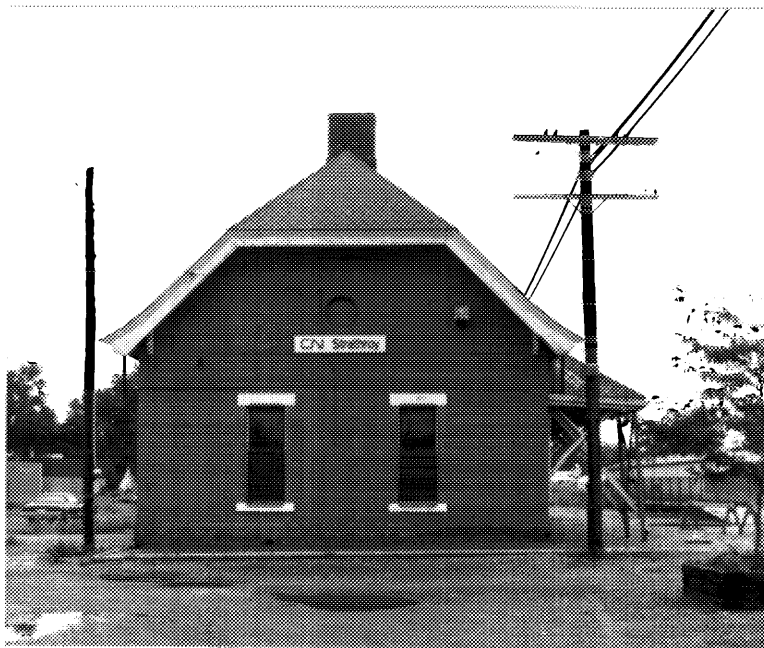
8 Strathroy station, west gable end. (Historica Research Limited, August 1992.)
