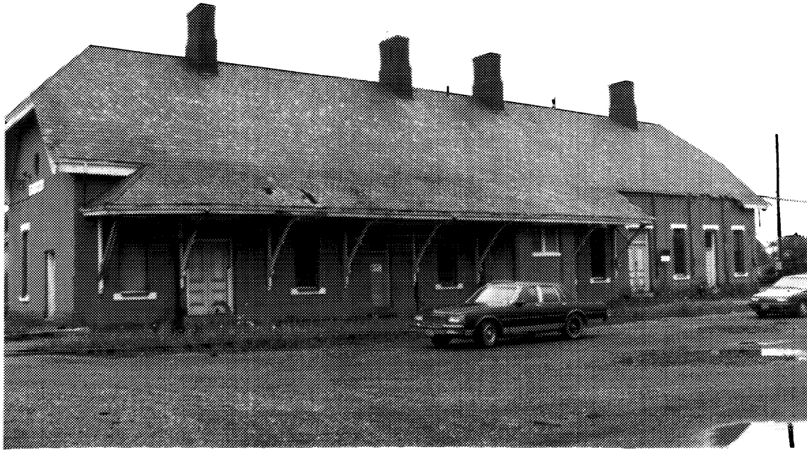
9 Strathroy station, north elevation. ( Historica Research Limited, August 1992. )
