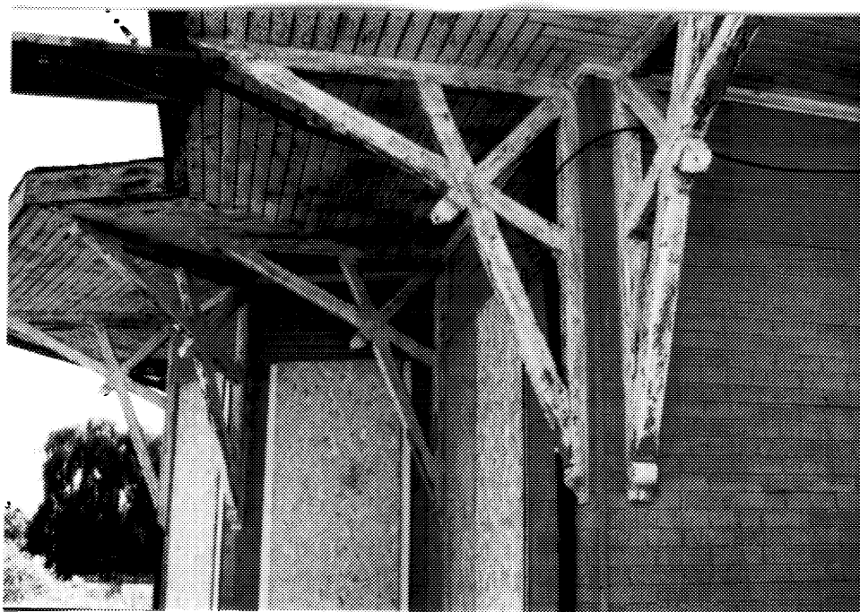
10 Glencoe station, detail of brackets, east end. ( A. M. de Fort-Menares, 1995. )
