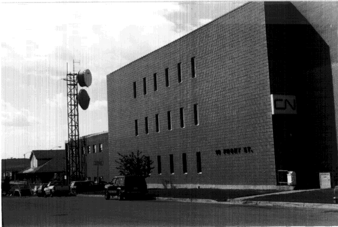
11 Office addition, town (south) side, Capreol terminal. ( M. Carter, Heritage Research Associates Inc., 1995. )
