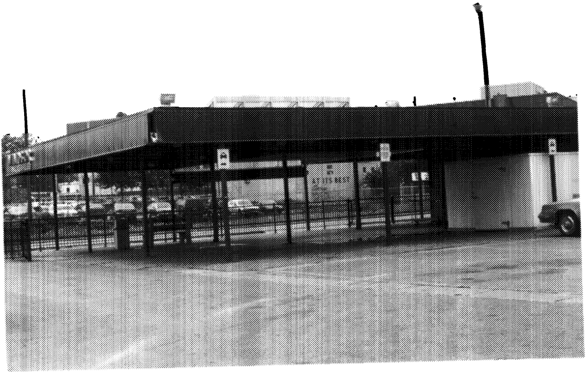
7 Windsor station, canopy shelter. ( Heritage Research Associates, 1995. )
