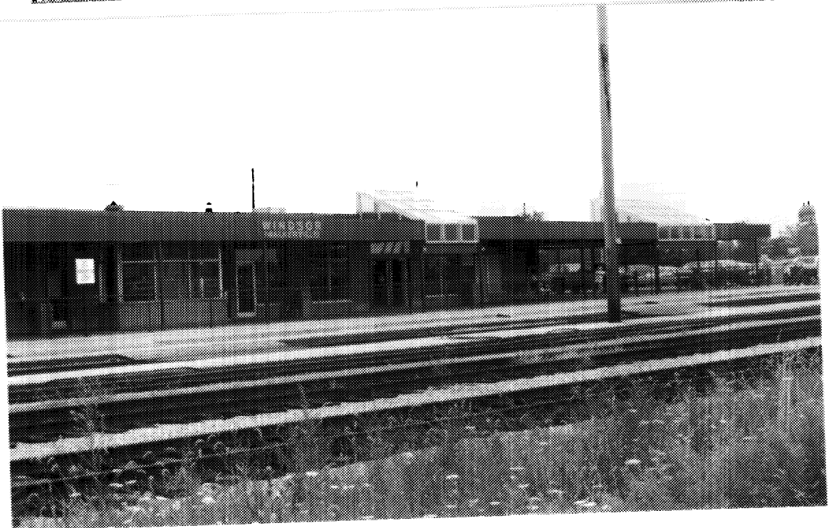
5 Windsor station, skylight structures. ( Heritage Research Associates, 1995. )
