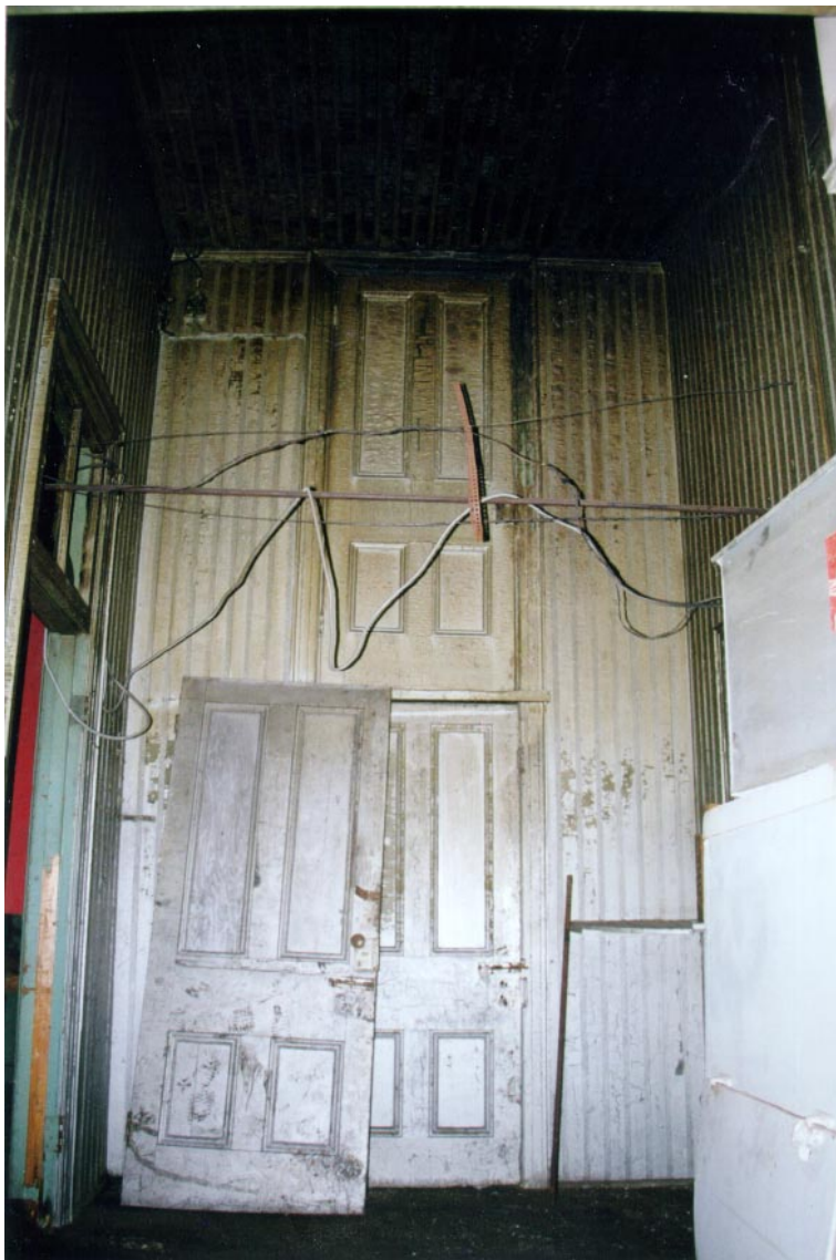
14 Former CNR station, Hespeler [Cambridge], interior hallway. (Murray Peterson, 1997.)
