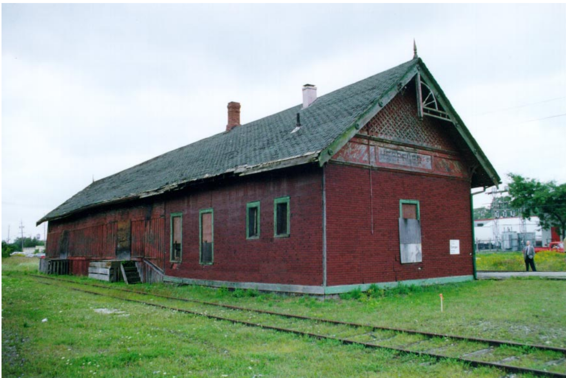
10 Former CNR station, Hespeler [Cambridge], east and town-side (south) facades. ( Murray Peterson, 1997. )
