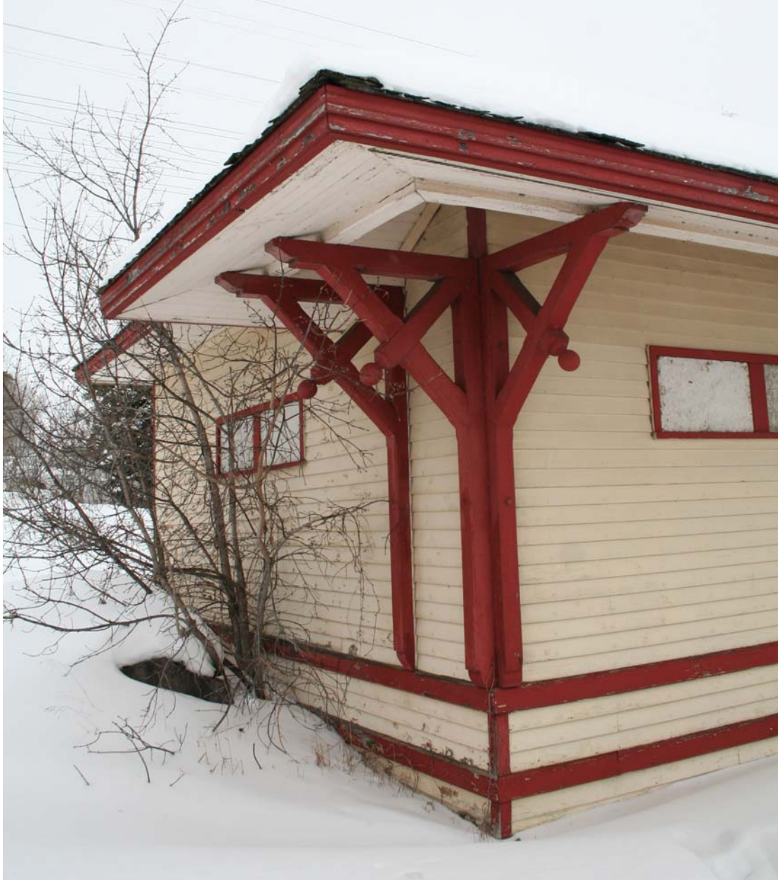
10 Former CNR/NTR station, Minaki, Ontario, detail of brackets on the track side (south) façade. ( Murray Peterson, 2009 )
