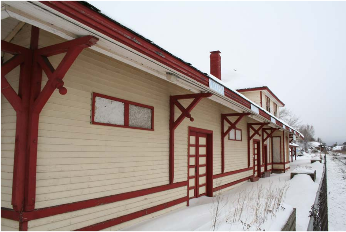
12 Former CNR/NTR station, Minaki, Ontario, overhanging eaves on the track side (south) façade. ( Murray Peterson, 2009 )
