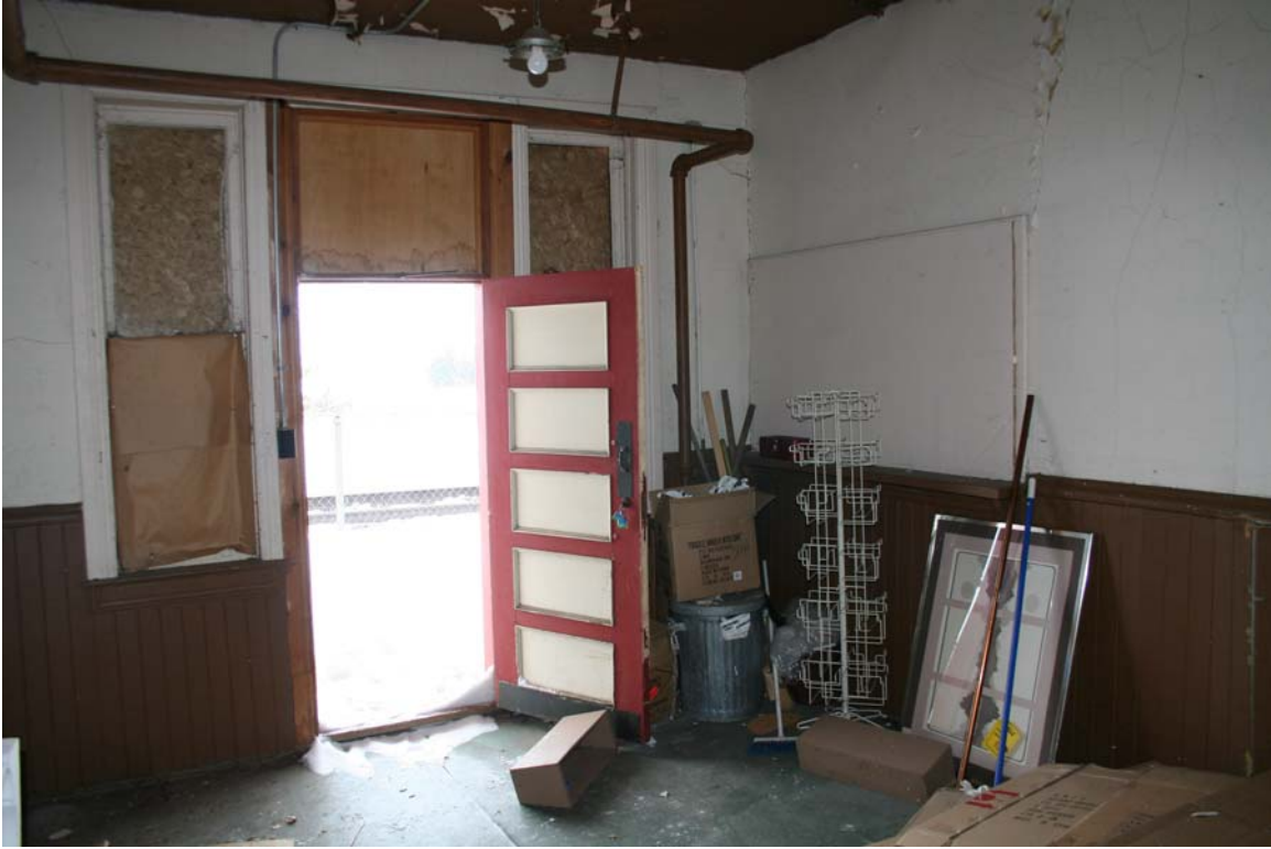
25 Former CNR/NTR station, Minaki, Ontario, front (trackside) doorway of the waiting room with ticket counter. ( Murray Peterson, 2009 )
