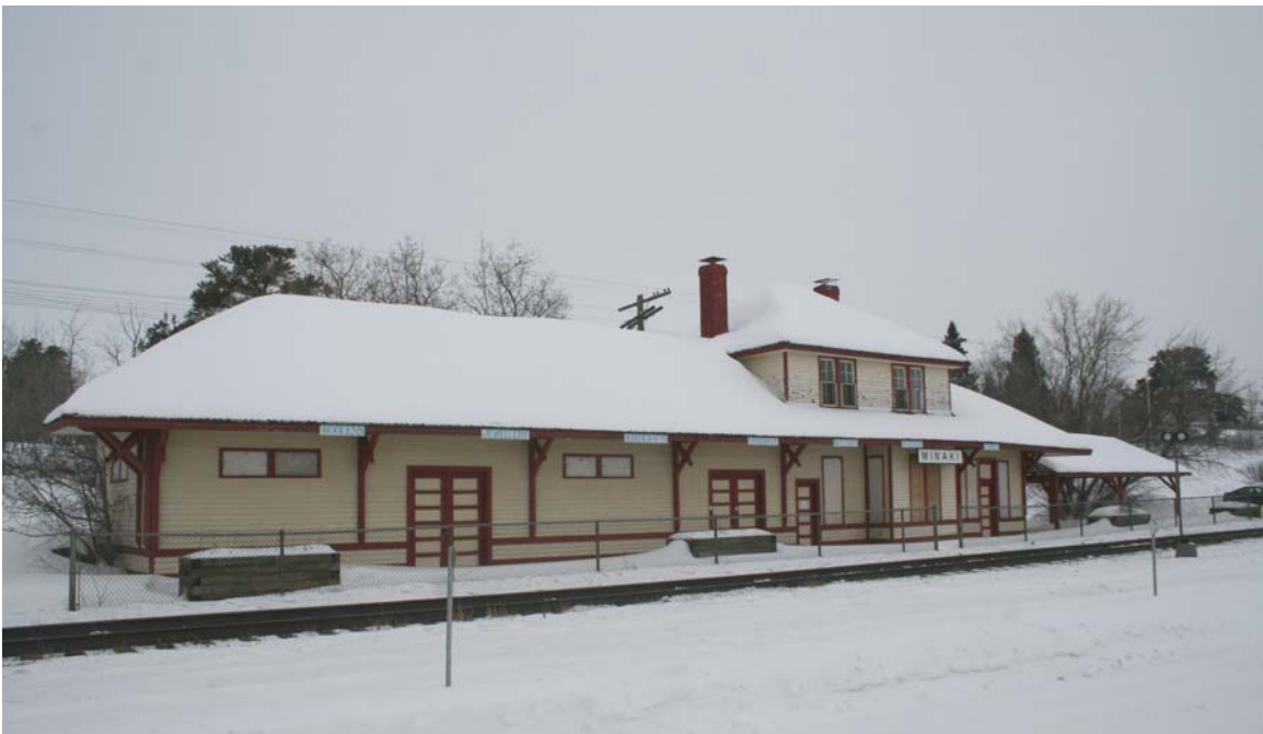
15 Former CNR/NTR station, Minaki, Ontario, track side (south) and west façades. ( Murray Peterson, 2009 )
