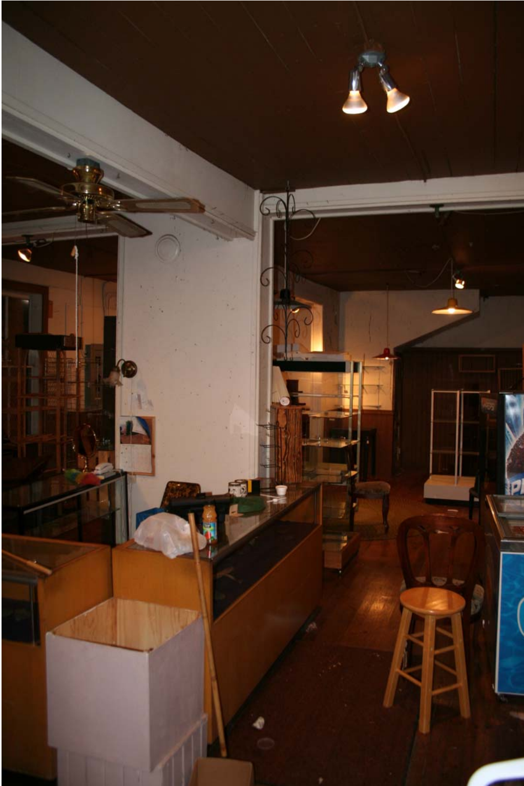
21 Former CNR/NTR station, Minaki, Ontario, looking east through the original office area. (Murray Peterson, 2009)
