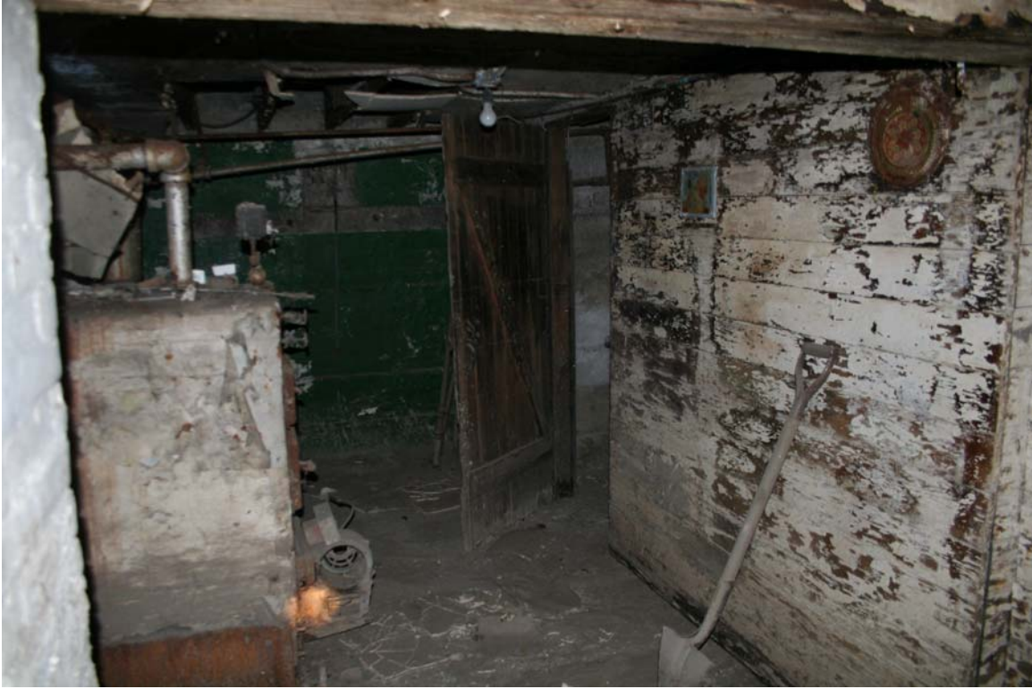
27 Former CNR/NTR station, Minaki, Ontario, basement. ( Murray Peterson, 2009 )
