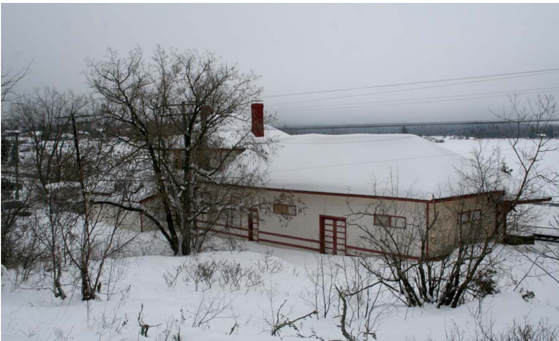
13 Former CNR/NTR station, Minaki, Ontario, town side (north) and west façades. ( Murray Peterson, 2009 )
